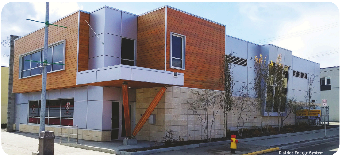
District Energy System
